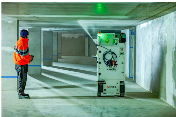
Painting robots can solve some of the labour shortages: Here the PaintBuddy from Caparol in action (Photo: Caparol)
